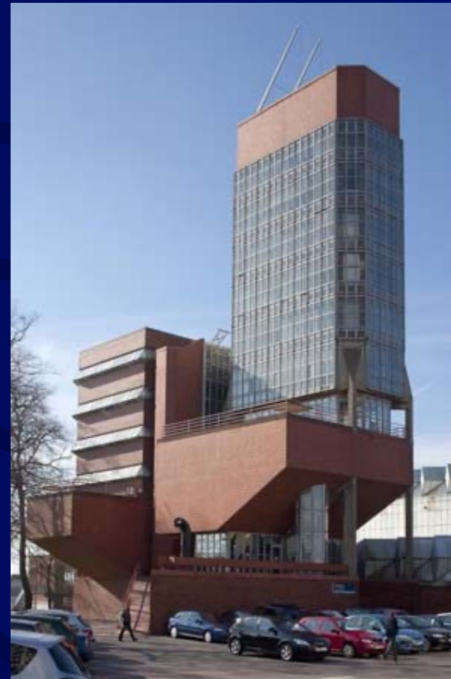
James Stirling, Leicester Engineering Building
